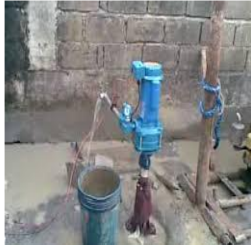
(B) Deep well drilling
