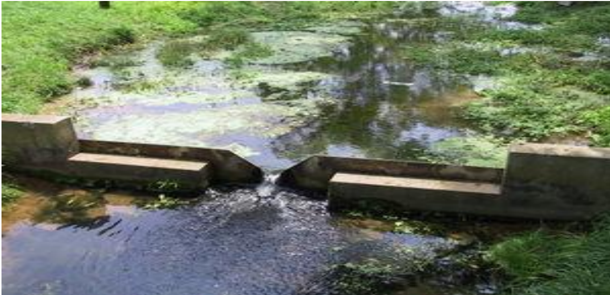
Figure 55: An example of a V-notch weir
