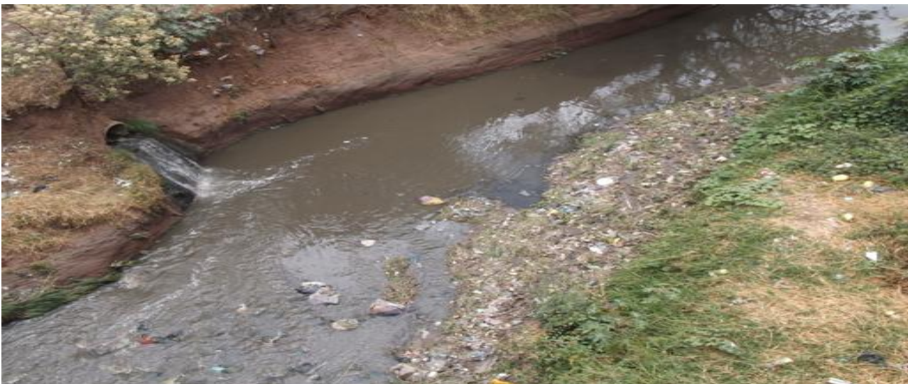
Figure 38: The effect of poor sanitation: liquid wastes are discharged into rivers and streams that may be used as a water source.
