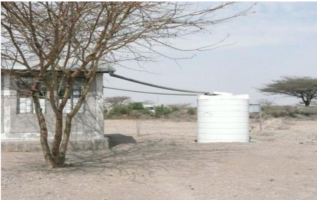
Figure 6: Rainwater is collected from the roof of this rural health post and stored in a covered, watertight Cistern. (Source Wikipedia)
