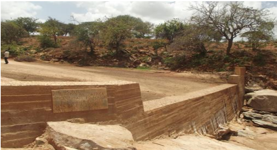
Figure 8: A sand dam in Kenya used as source of rain water collection
