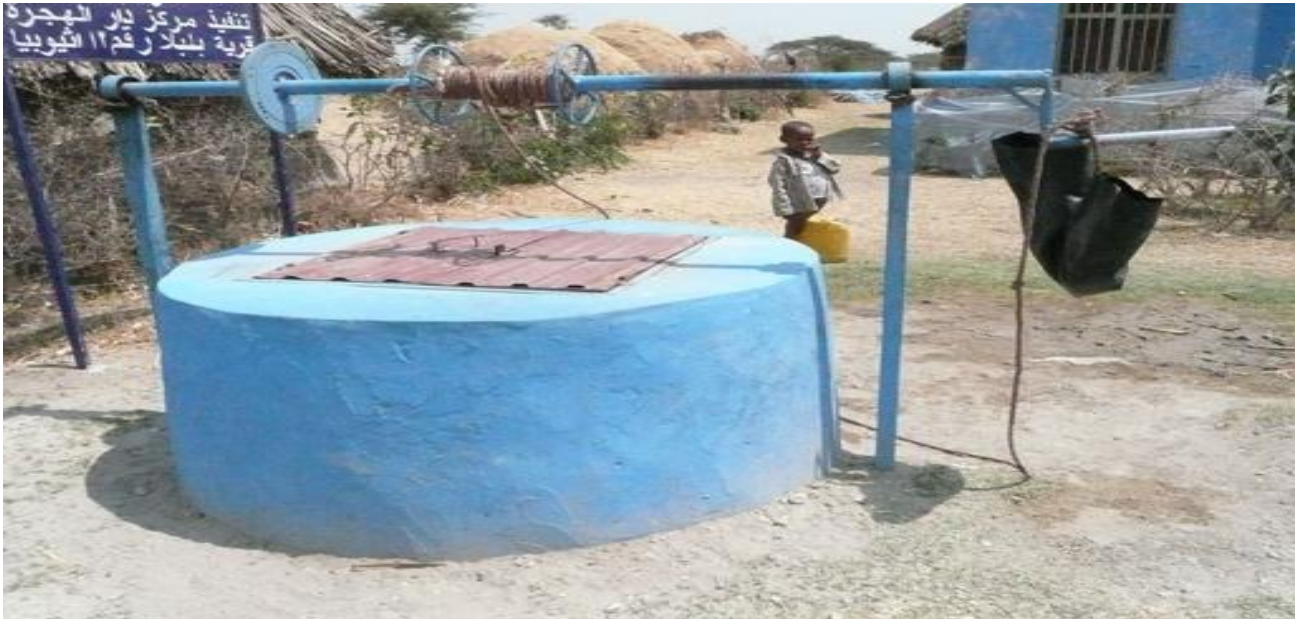
Figure14: Protected well with concrete surround and a lid. Note the black plastic bucket is suspended off the ground to keep it clean (source OWP, M5)
