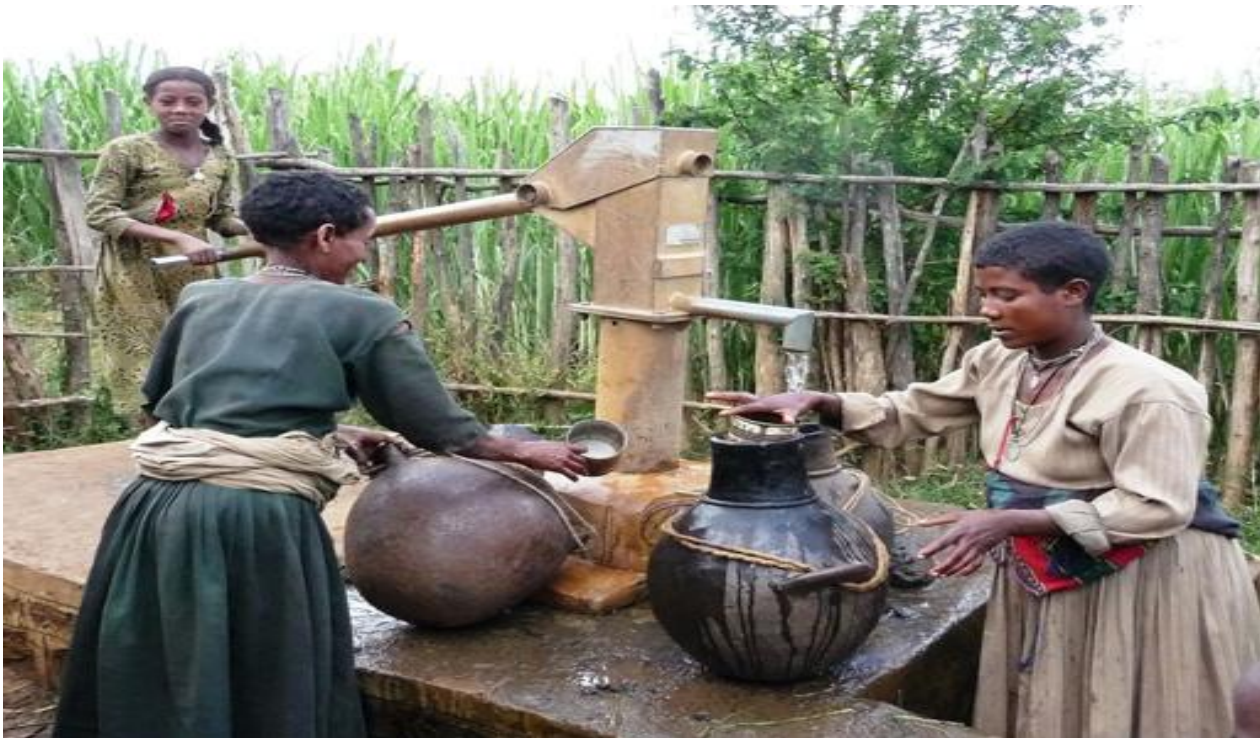
Figure13 Hand pump over a protected dug well. Note the concrete surround and the fence to keep out animals (source: SNV manual)
